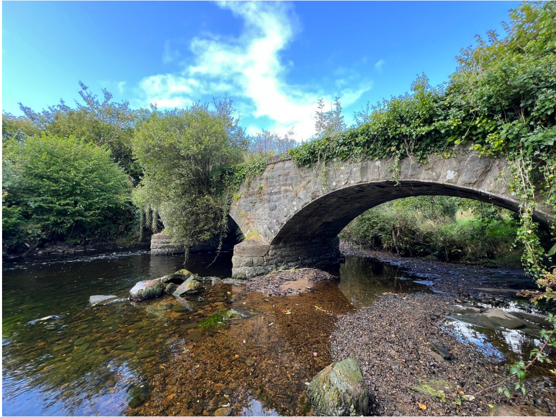
Photograph 8-4 - Existing Stone Arch Bridge at River Eske Crossing
