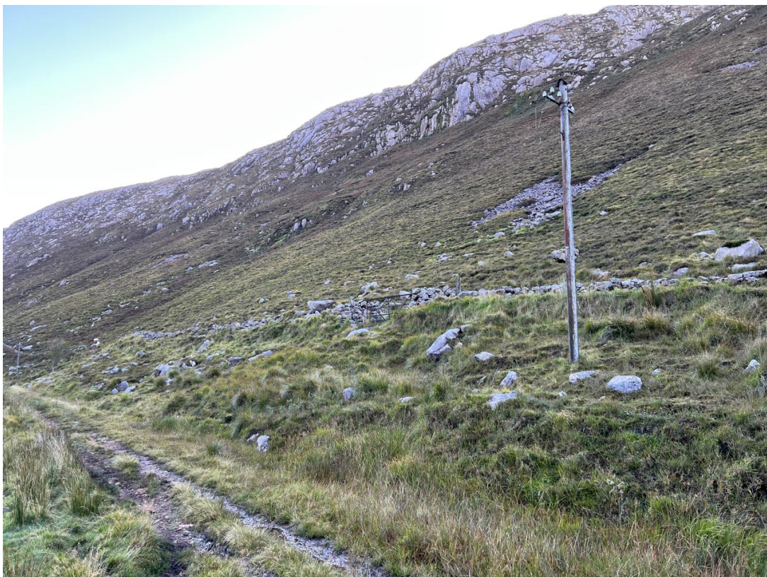
Photograph 8-8 - Existing Slopes at Barnesmore Gap (1)
